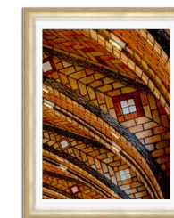
4th Floor - Elevator Lobby West Side Market Ceiling
