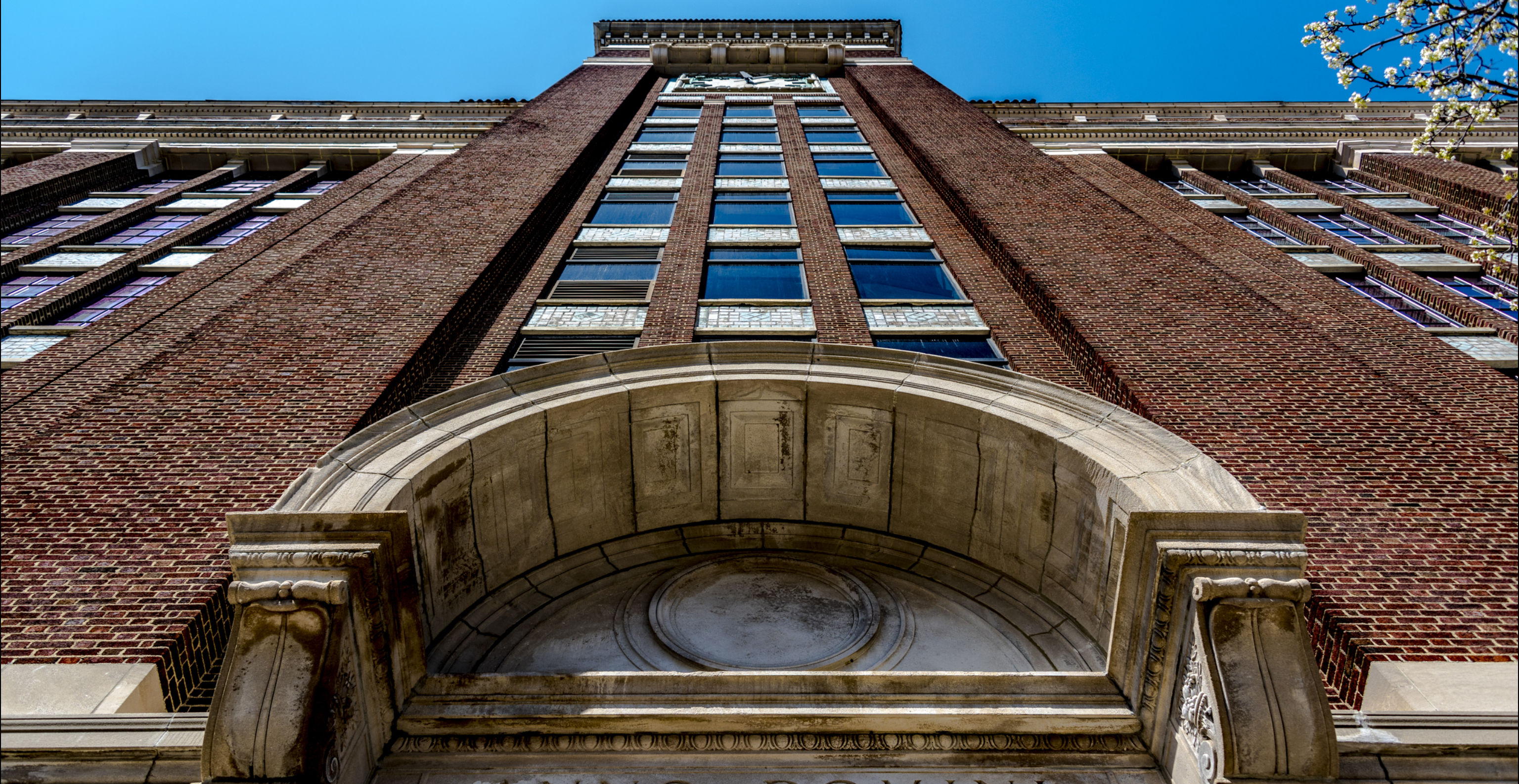
THE BALDWIN PIANO BUILDING CINCINNATI, OH
